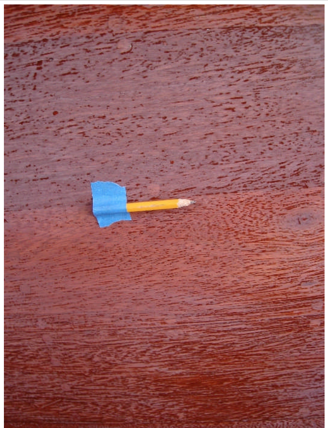
Topside boards after more sanding are ready for cleaning and varnishing. The surface tension depressions are few and small.
